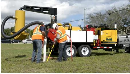
**To ensure no underground interference. Once the Locates are done by first call all underground utilities will be daylighted via hydrovac**
