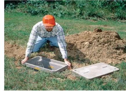
**Hand Holes will need to be placed to accommodate the splice enclosures throughout the network.**
