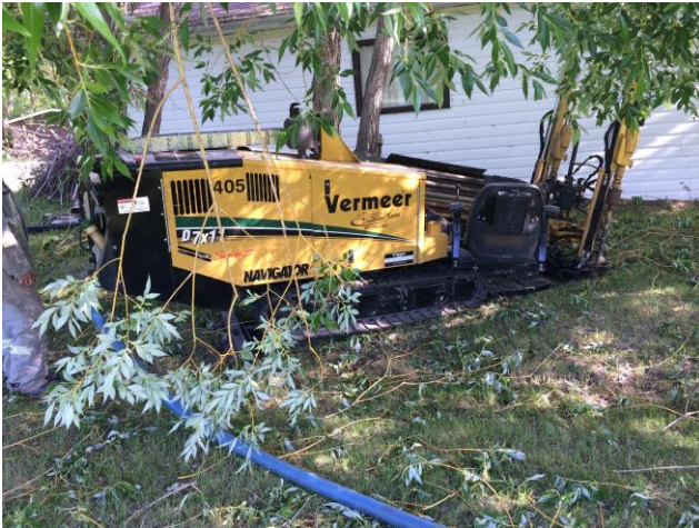
Directional drilling for service connection
