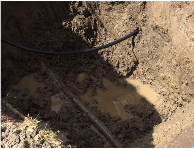
Pulling in service line after drilling
