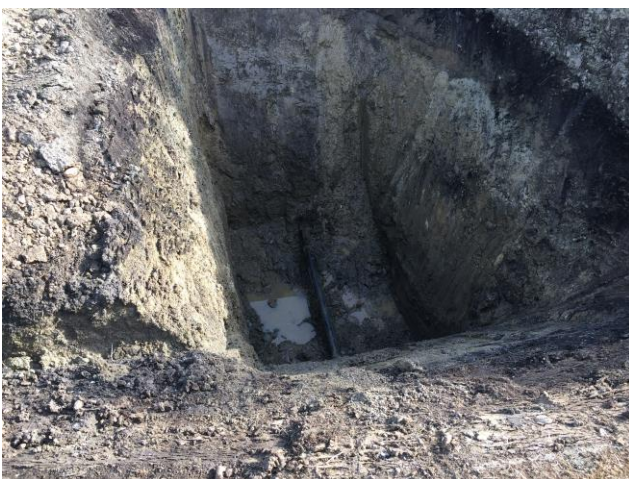
Main line exposed
